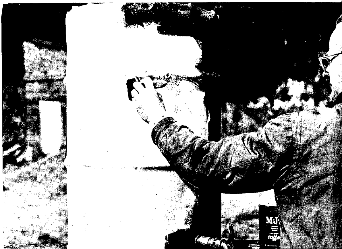
22. LET BARREL DRY, THEN PAINT OUTSIDE WITH ALUMINUM PAINT
