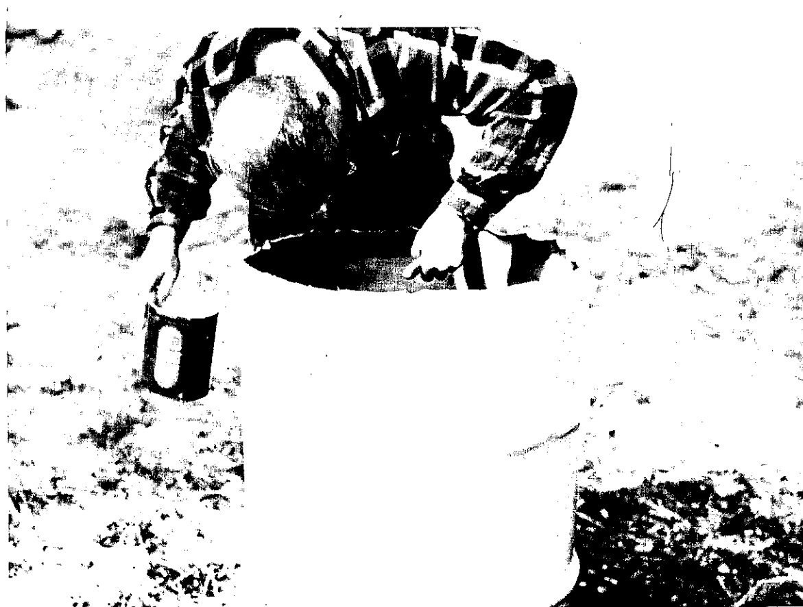
23. PAINT INSIDE WITH ALUMINUM OR ASPHALT PAINT
