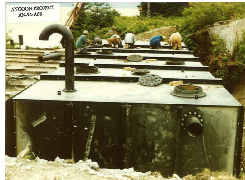
Angoon Settling Tanks
