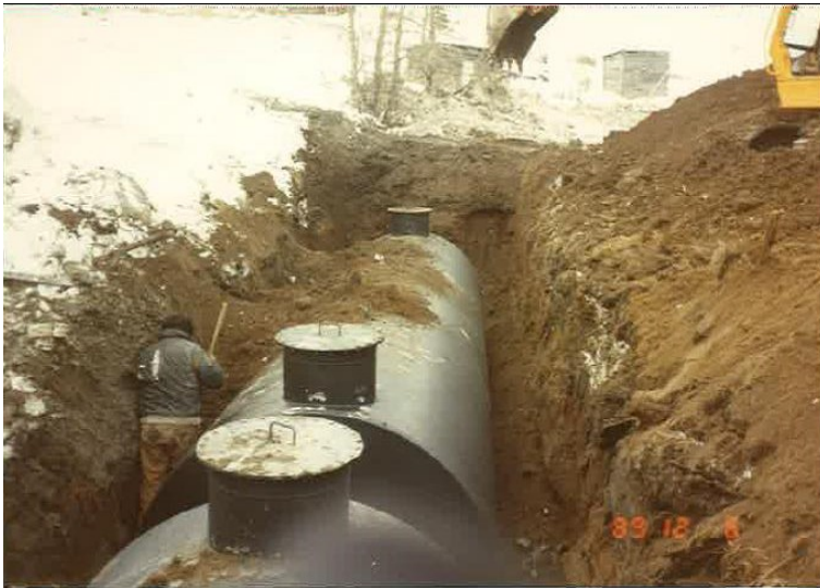
Tyonek Settling Tanks
