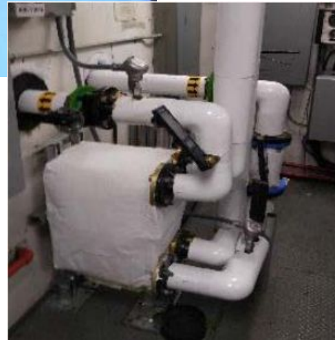
Water jacket heat recovery
