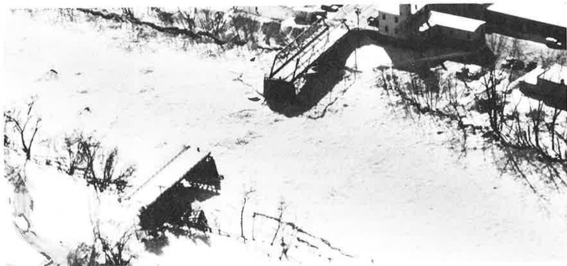
Bridge on White River, Vermont, collapsed during January 1990 thaw.
