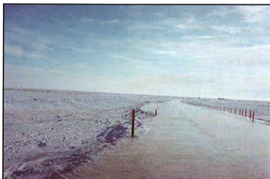
Ice road. Travel across the open tundra with heavy equipment for oil exploration is restricted to winter, when seasonal ice roads can be created.
