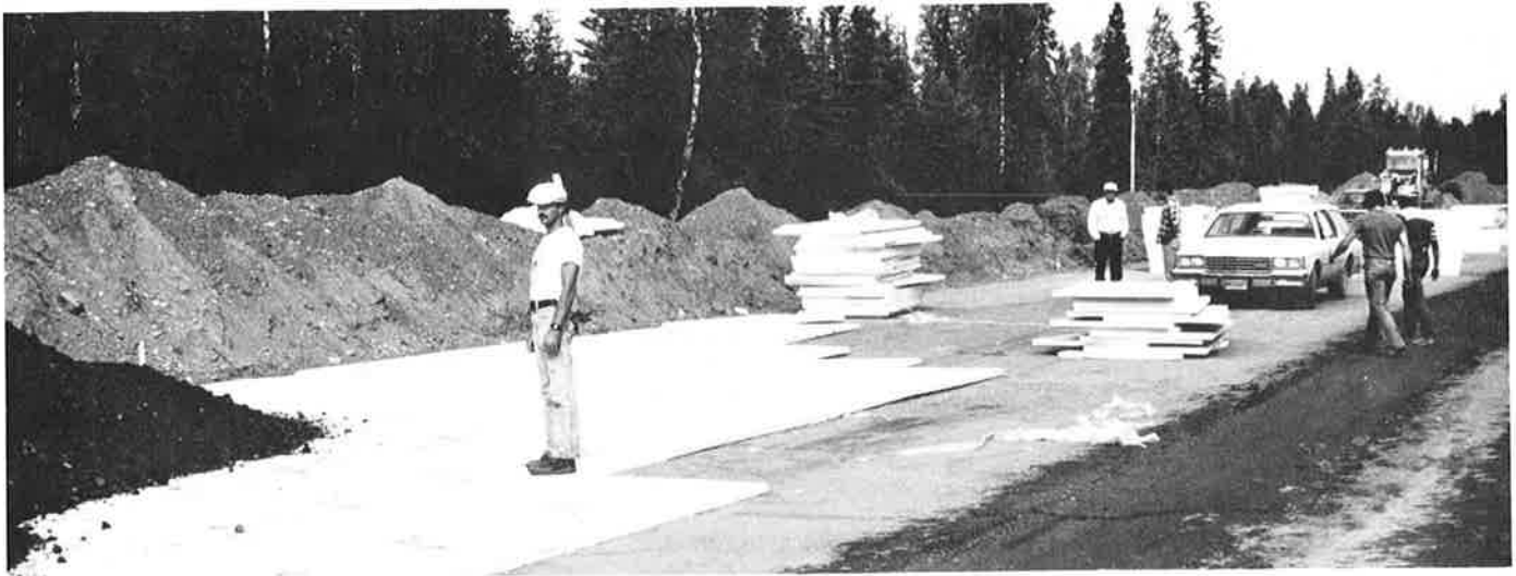
Experimental insulation being installed to control thawing of permafrost underlying a highway.
