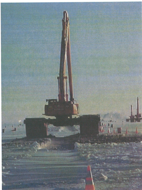
Enormous backhoes with significant reach used on strengthened ice to install an offshore pipeline in the Beaufort Sea.
