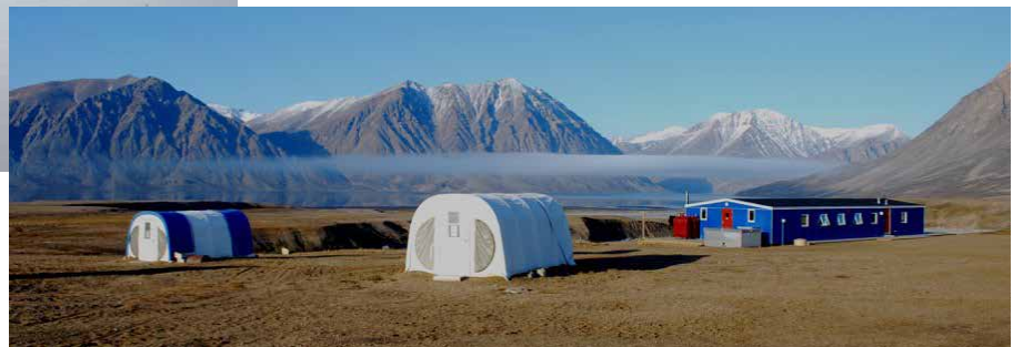
(BELOW) The Zackenberg Research Station, in Northeast Greenland, has nine houses, a powerplant, waterworks, and an airstrip. Photo credit: Morten Rasch
