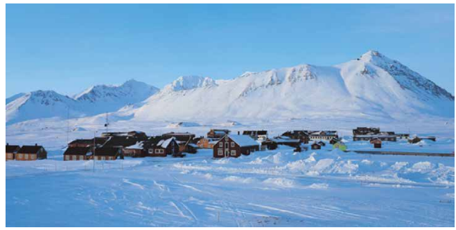
Overview of the Arctic Dasan Station. Credit: KOPRI
