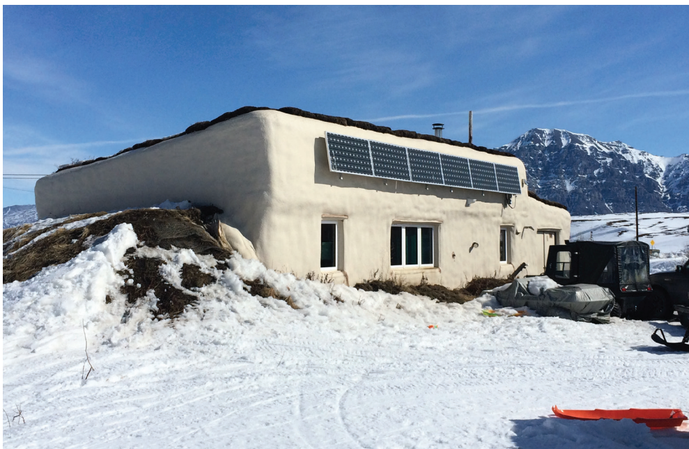
FIGURE 3. The CCHRC demonstration home in Anaktuvuk Pass, Alaska. Photo by USARC
