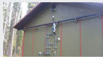
Rainwater catchment, intake and water overflow pipes, and waste water outlet.
