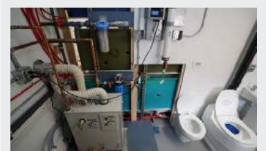
In-wall water storage tanks, drinking water filters, and a low-flow or dry toilet option.
